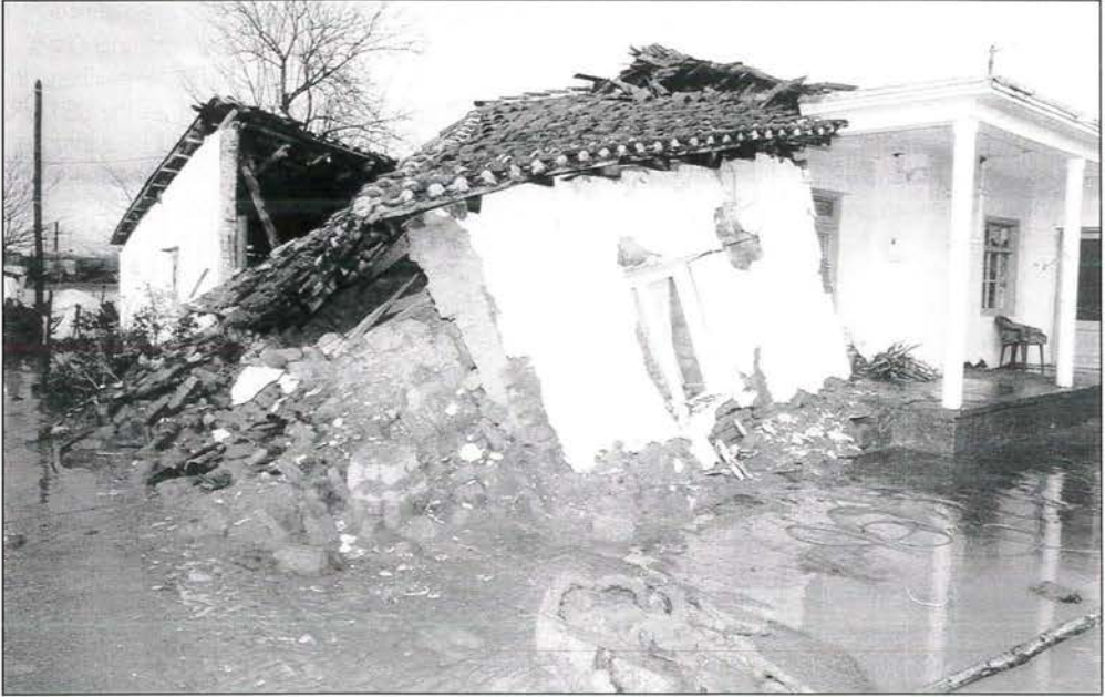
Severe thunderstorms at Xanthi, Greece, on 30 November 1996, caused floods with the loss of three lives, havoc in rural areas and extensive damage to buildings, railways and roads; power and water supplies were cut off.
